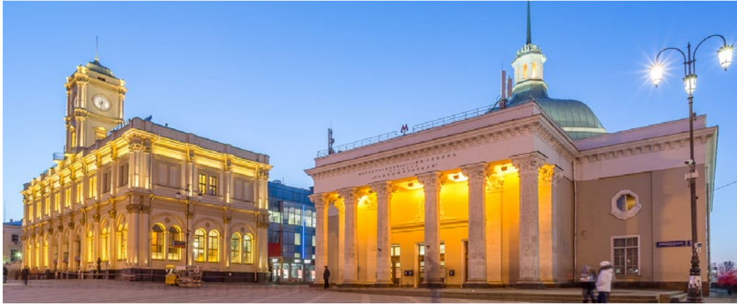
Rolling stock acquisition, carriages
